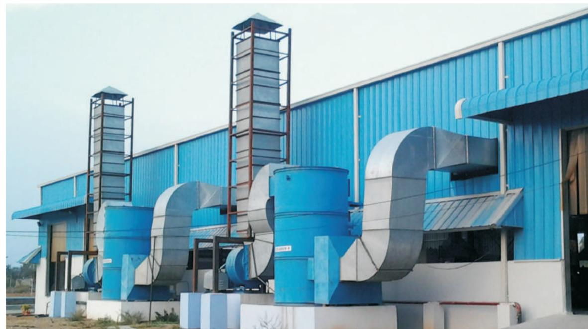
**UK Engineering Projects** have an established expertise in wet scrubbers. Scrubbers remove both particles and gases from exhaust stream of many industrial processes.
