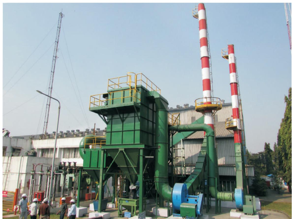
**UK Engineering Projects** bag filters are automatic air cleaning system. Pulsing jet of air is used to remove dust from bags supported by metal cages.
